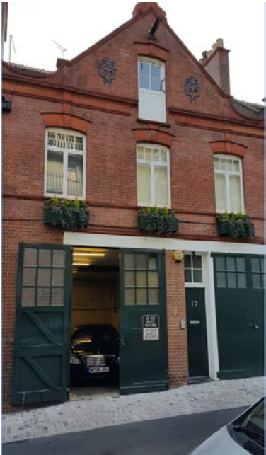
12 Bourdon Street Front Elevation (Door Open)
