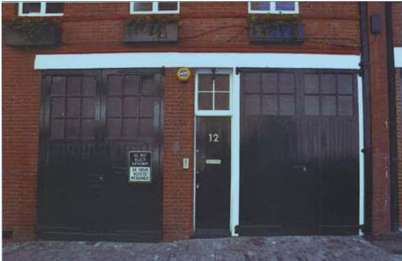
12 Bourdon Street Front Elevation (Door Closed)
