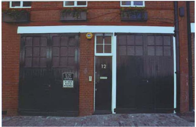
12 Bourdon Street Front Elevation (Door Closed)
